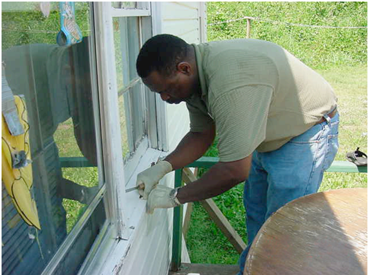
Regional Environmental Health Specialist Warren Richardson checks a Chatham County home for potential lead paint hazards.
